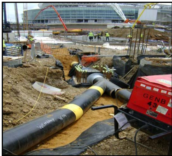
Photo 2: Envac pipes being laid at Wembley City
