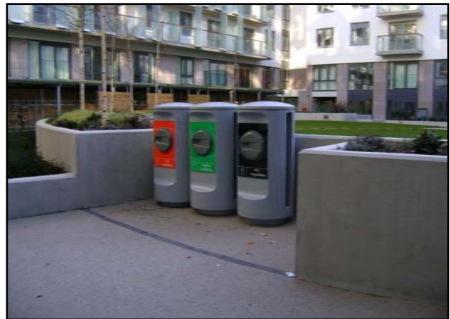
Photo 1: Inlet Chutes at Wembley City
